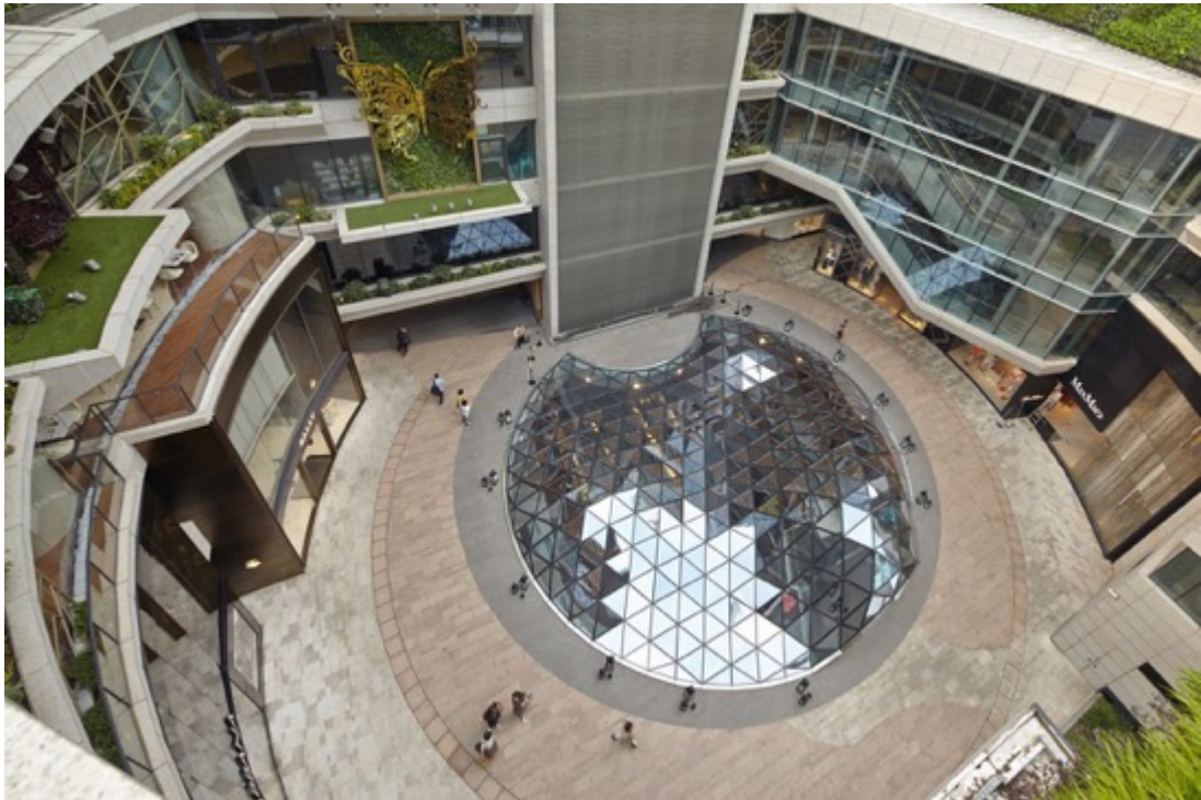
Figure 22. An aerial view of the inner courtyard of K11 (Sánchez, 2013).
