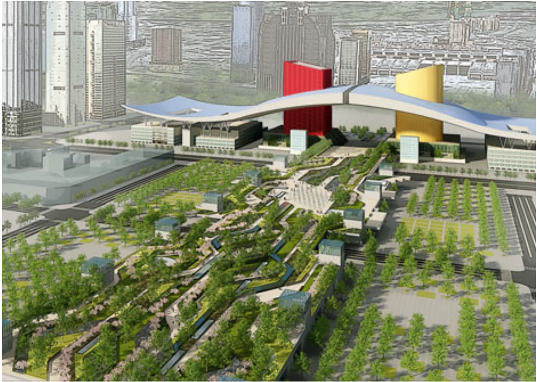
Figure 42. Shenzhen Civic Center at the Futian District, designed by SWA Group (Chalcraft, 2012).
