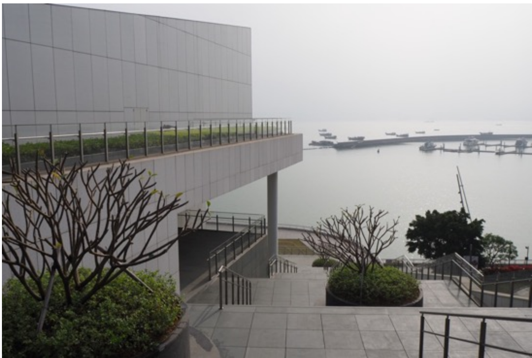
Figure 143. One of the grand stairways by the Waterfront Plaza entrance (own photo).
