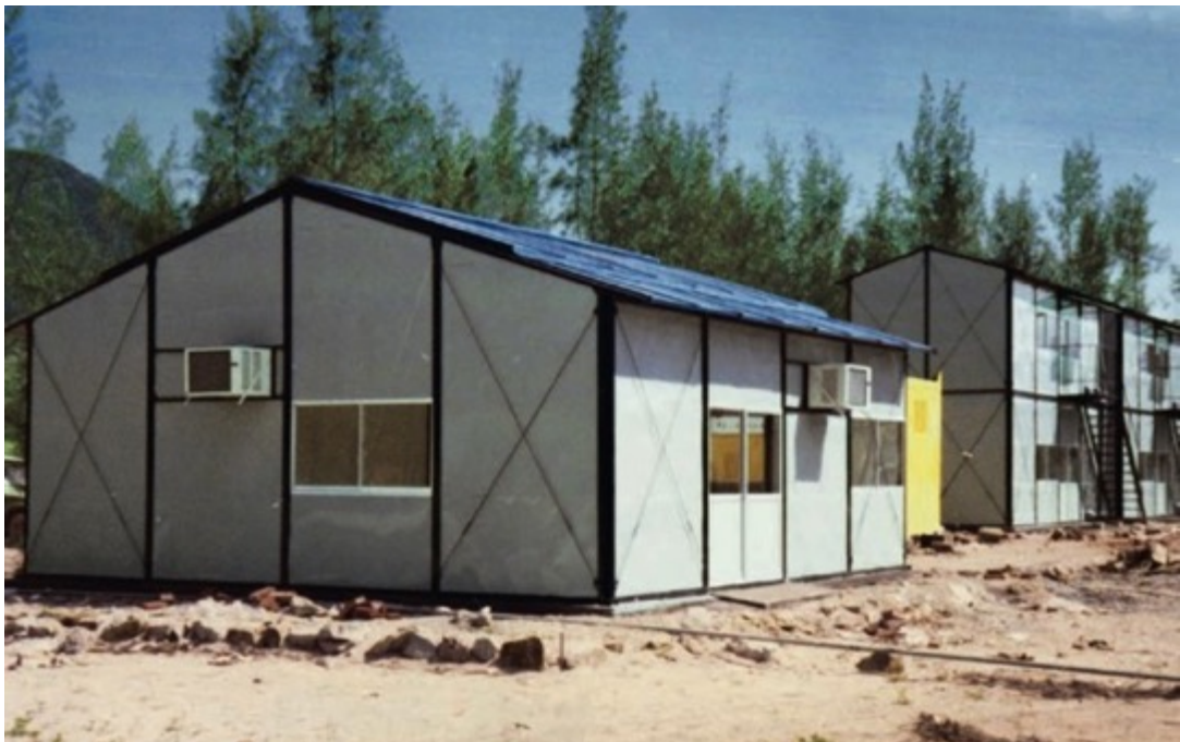
Figure 166. The corrugated metal office CMSK used as headquarters in 1979 (ibid., p.54)
