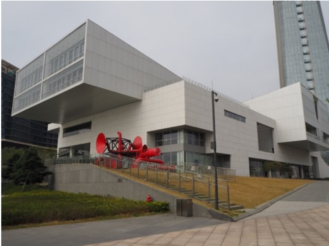
Figure 79. Own photo of the SWCAC taken from the waterfront route (South elevation).
