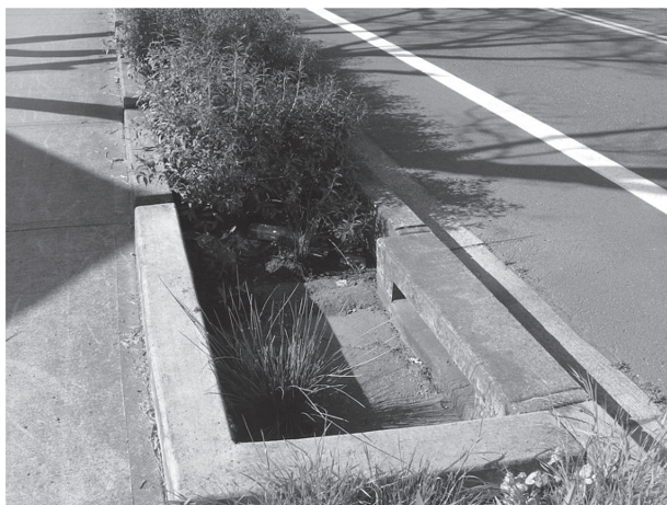
Figure 1 Incomplete bioswale showing water inlets.
