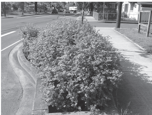
Figure 3 Bioswale extending into the road.
