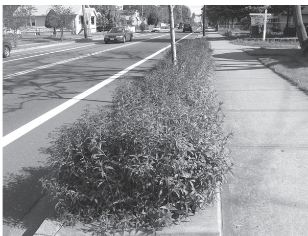
Figure 4 Bioswale not extending into the road.
