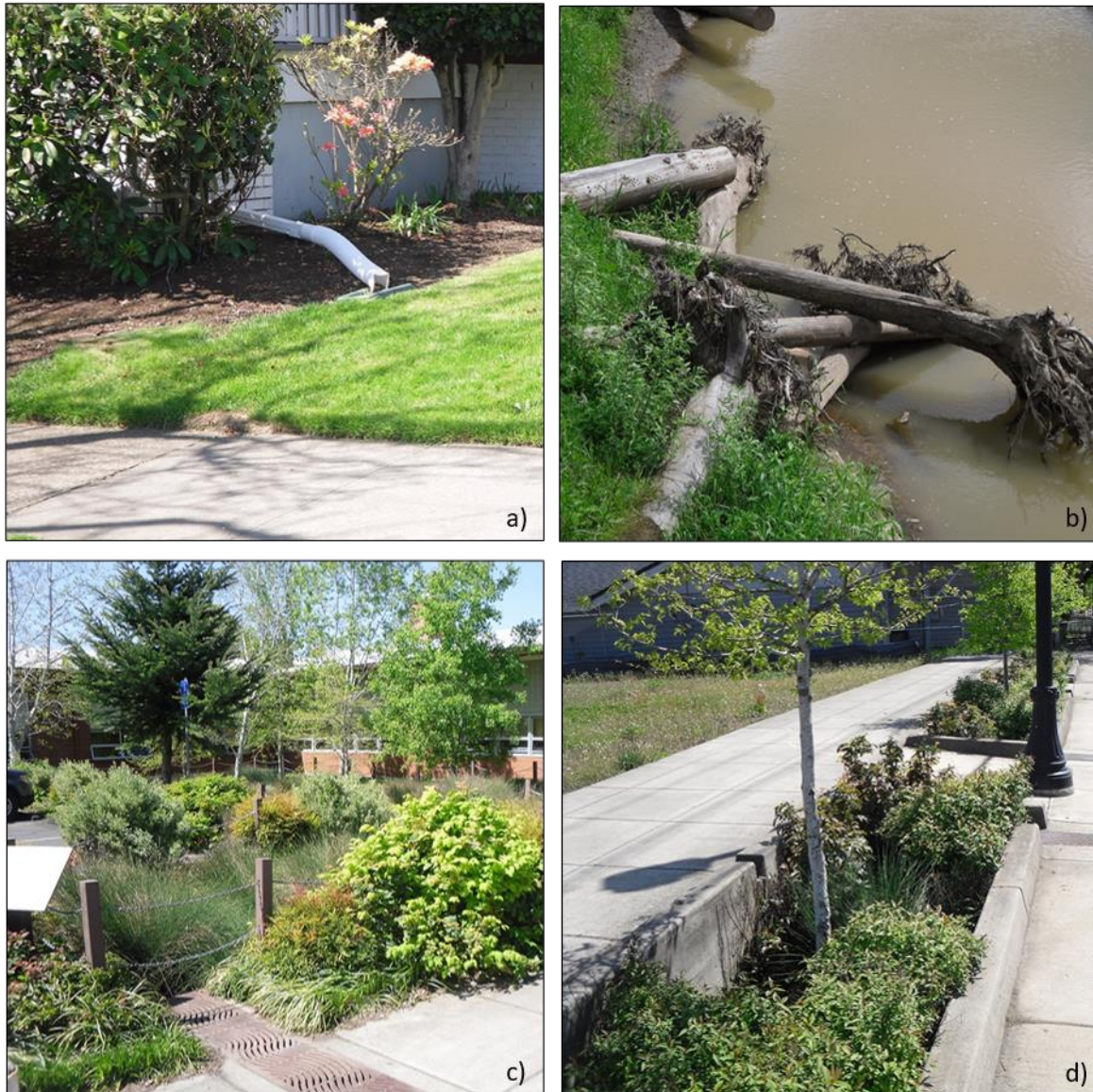
Figure 2. Blue-Green Infrastructure (BGI) and stream restoration activities in Portland. a) Downspout disconnection in a residential area of East Portland, b) large wood structure constructed in Johnson Creek as part of the East Lents Floodplain Restoration Project, c) rain garden at Mount Tabor primary school, d) typical green street bioswales. (Photos: E. O'Donnell, April 2013 (a, c, d), May 2014 (b)).
