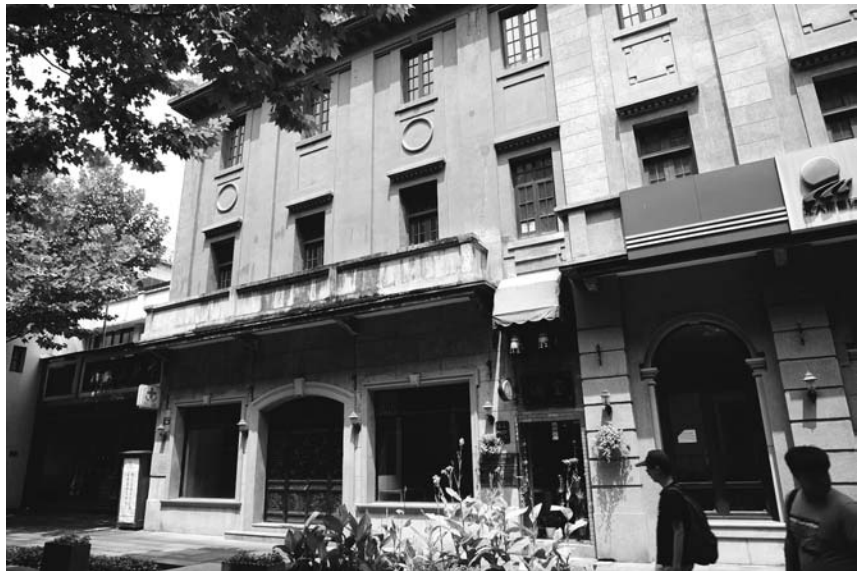
Figure 11 The former premises of Wuzhou medicine shop, built in the 1920s, preserved and renovated on Southern Song Imperial Street, Hangzhou (author's photo, 2014).
