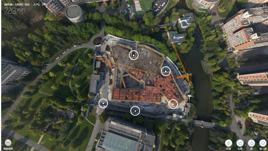
Figure 3.3. An Aerial View of the Construction Site.
