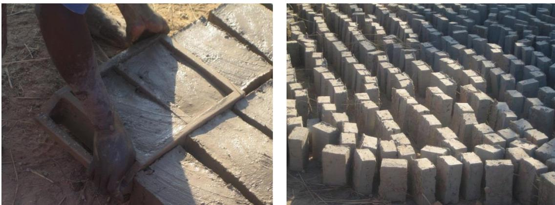
**Figure 11.** Adobe is one of the most environmentally friendly construction materials.
