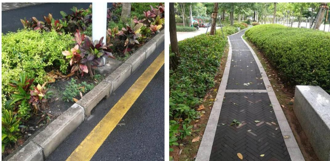
Figure 2.2 Bio-swales on roadsides (left) and permeable pavement (right) in Shenzhen
