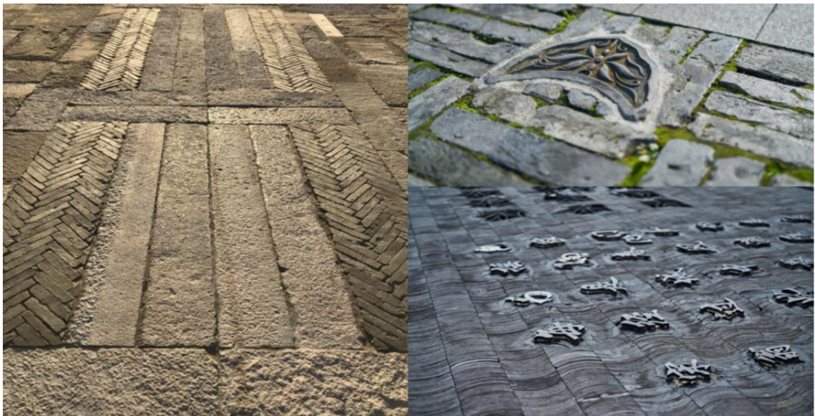
Figure 72 Use collected old materials to pave the road.
