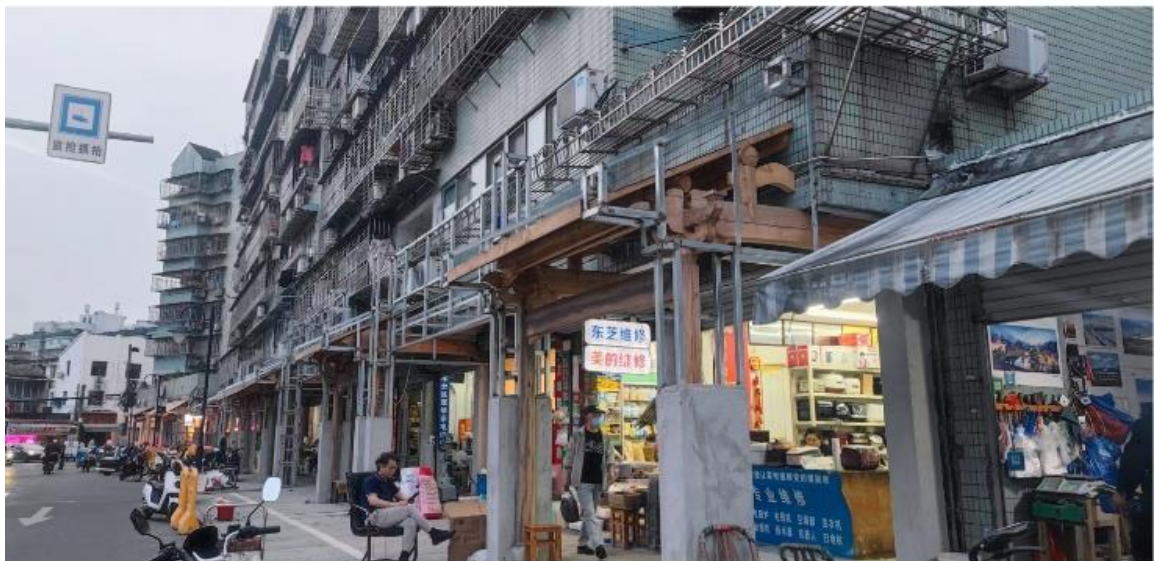
Figure 120 The under constructing façade renewals for old multi-story apartments in Xianhou Lane.
