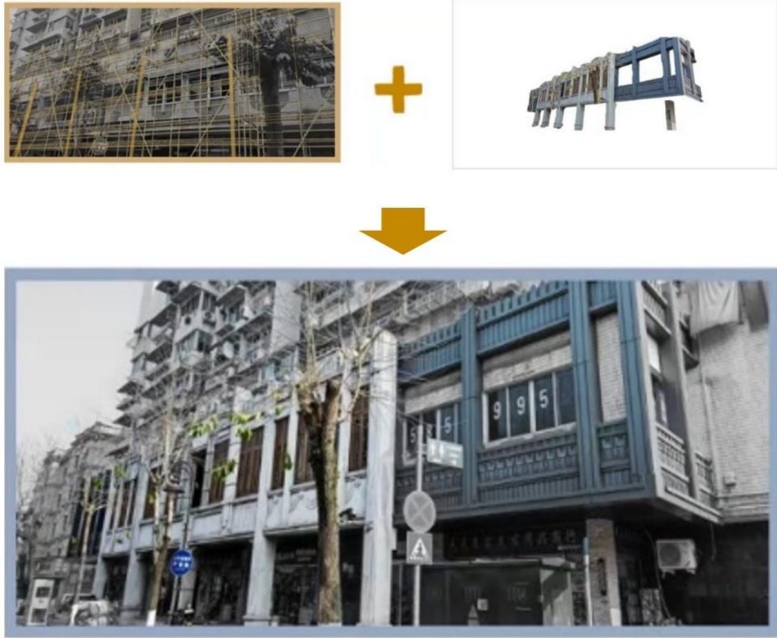
Figure 121 The attached façade on buildings along Jiefang Street.
